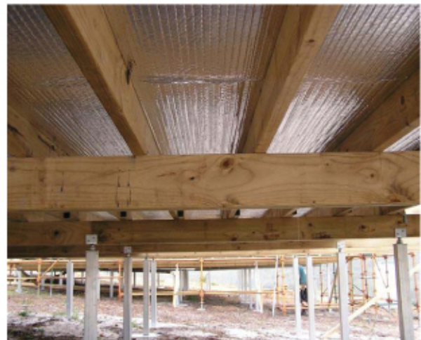
Installed over floor joists
