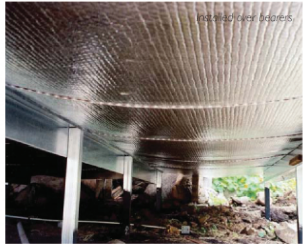
Installed over bearers
